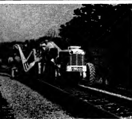
LAYING WELDED RAIL
